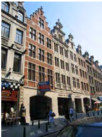
Rue de la Montagne n°s 24 to 40 - block 6 pastiche architecture
