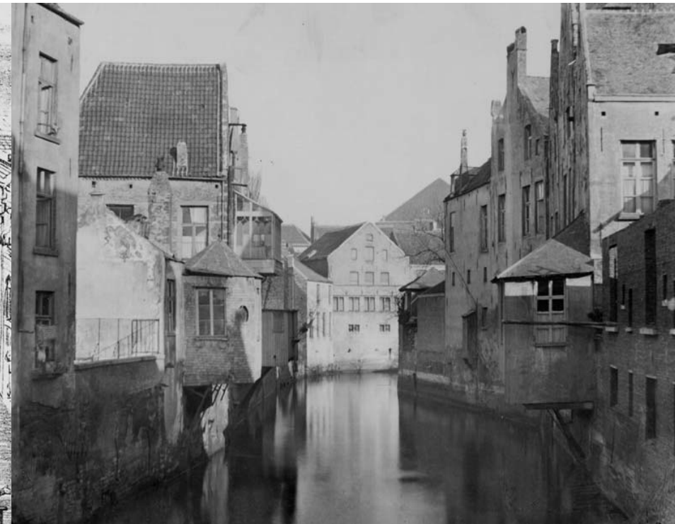
The River Senne looking downstream from Vanniers bridge (1867) Archives of the City of Brussels
